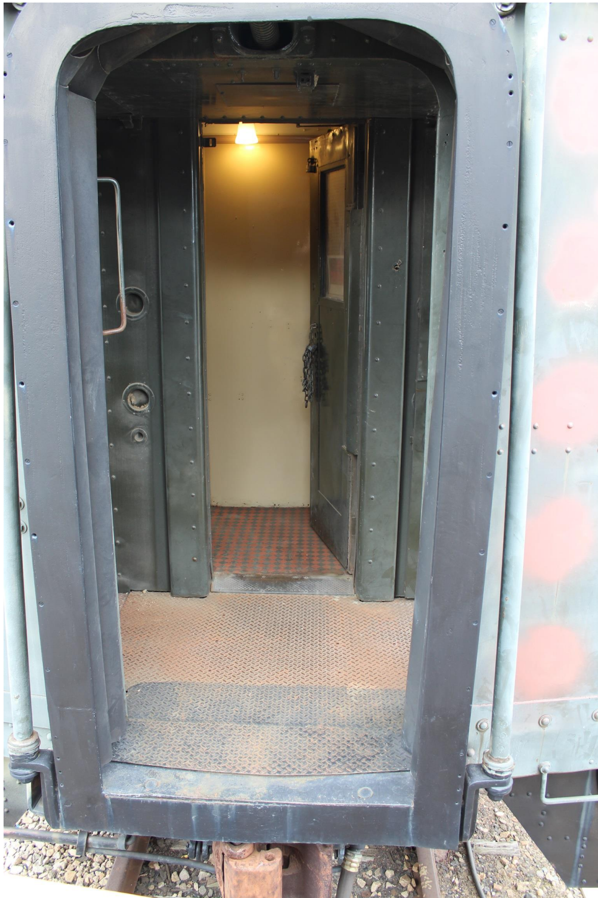
Entry hallway and vestibule platform on the Men's room end of the car. The red/black check flooring is the original from 1911. Steel grid plate installed on the platform to replace the open grid roof walk used during MOW. Buffer plates added in 1997. Buffer curtains fabricated and added in 2001.
