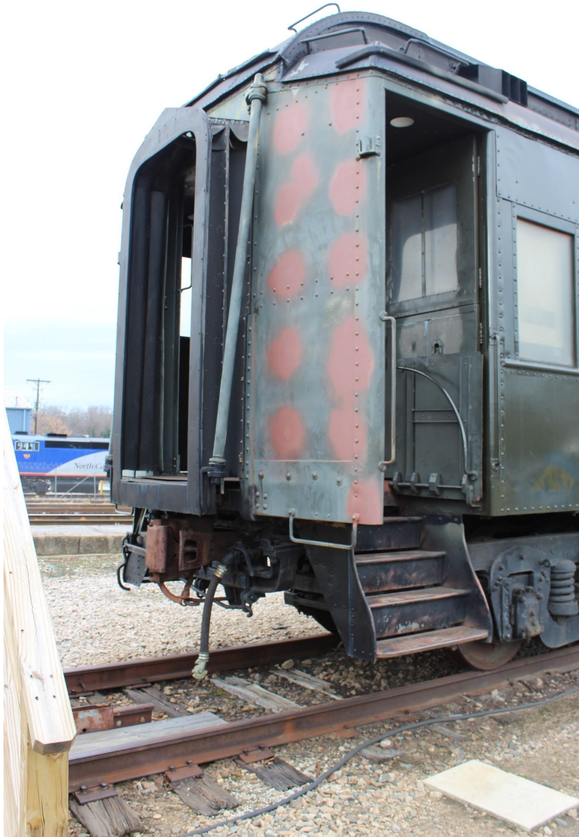
Vestibule on Men's room end of the car. The primer spots are where grab irons had been in place from MOW days. The holes have been welded shut and awaiting new paint.
