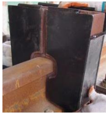
Sand type with sealing groove, easy to seal the box
