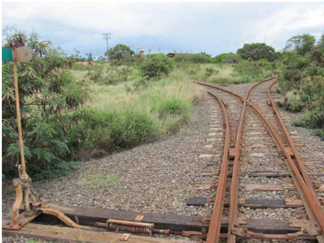
Spring Switch and Turnout – Puukolii – North Leg of Wye
