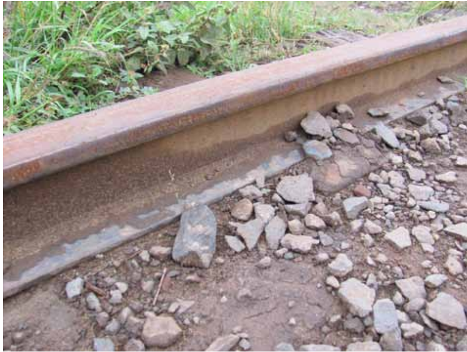
Typical section of 60AS Rail in good condition
