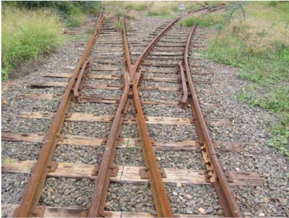
Typical #6 Right Hand Turnout – Puukolii Yard
