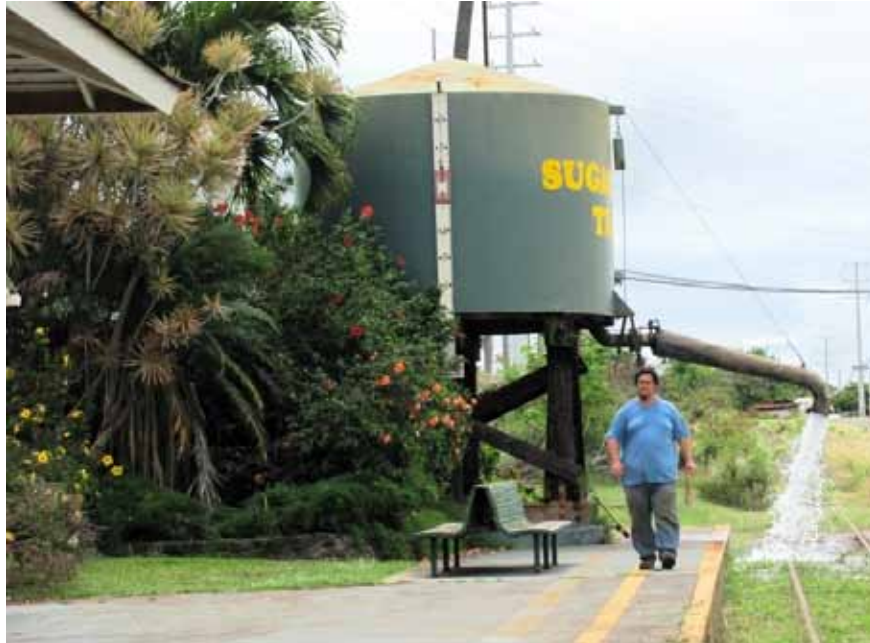
5800 gallon Water Tank and Spout for fueling steam locomotive tenders
