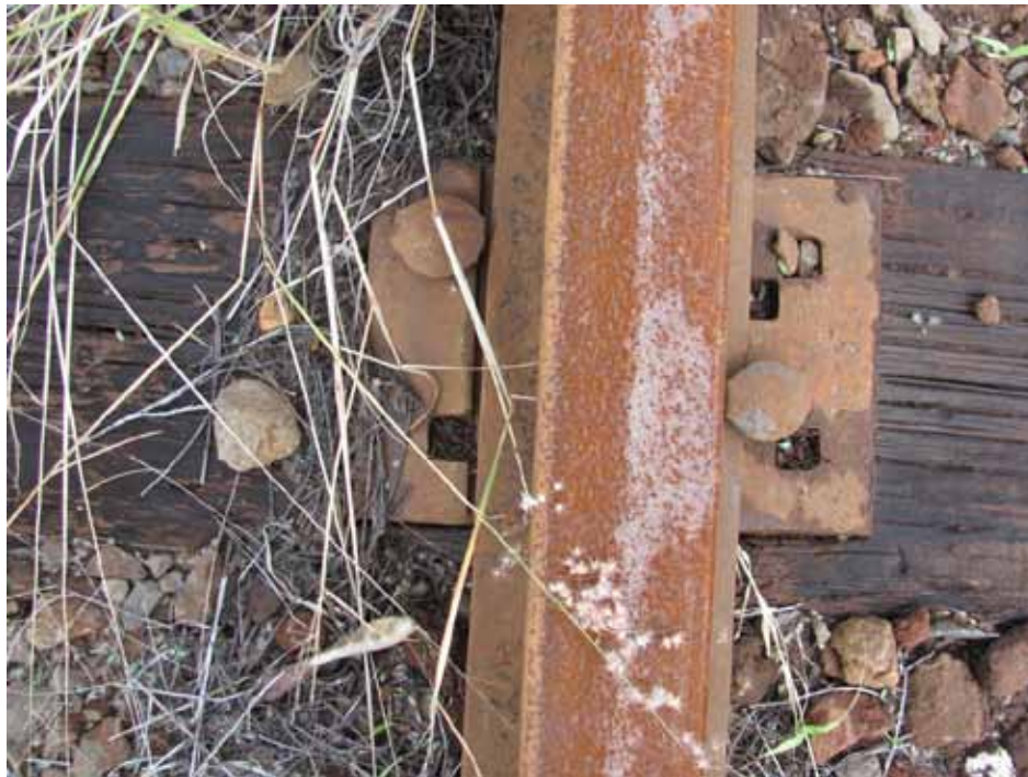
60AS rail with typical 6"x8" plate and spike pattern
