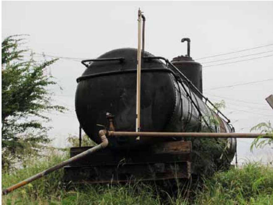
3100 Gallon Reserve Oil tank – Old Tank Car
